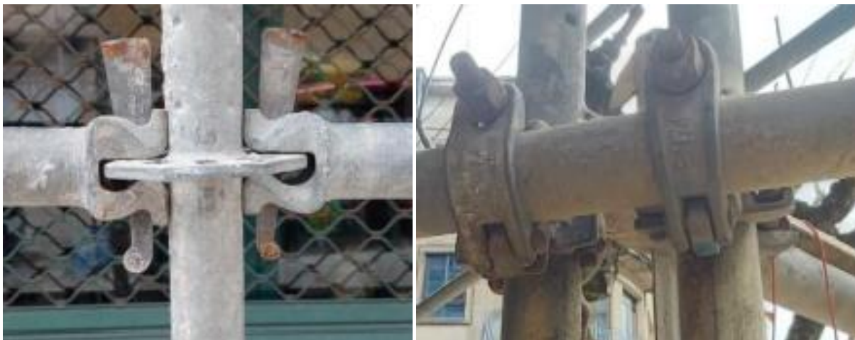
Gambar 4. Sambungan kunci cakram & quick round tube coupler (Cabaleiro et al., 2023)
