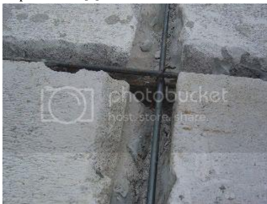
Gambar 4. Sambungan panel lantai [1]
